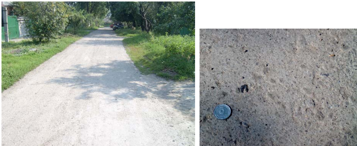
Fig. 4 General view of surface course from cold mixes based on milled asphalt concrete on composite binder after 8 months of service
